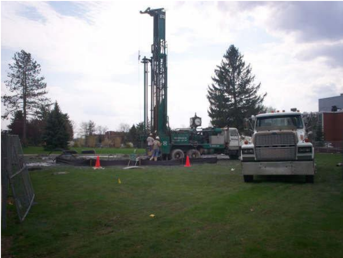
Figure 5: Drilling of a well-field, equipment shown to scale
