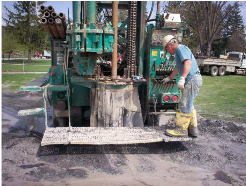
Figure 1: Workers drilling a well to pipe into the geothermal reservoir
