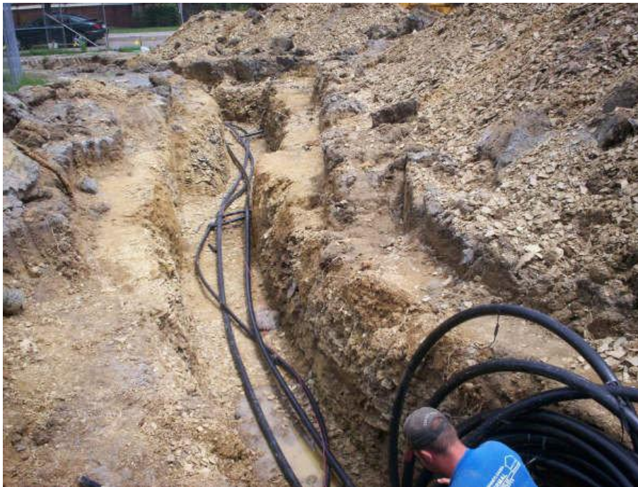
Figure 3: Pipe installation in progress
