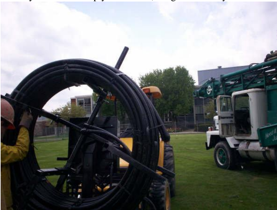
Figure 2: pipe "loop" ready to install
